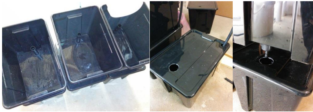
Figure 6 From left to right: Adding the bulkhead fitting & standpipe to the grow bed component, drilling the bulkhead fitting hole and pump hose in the support lid of the grow bed, and a close-up of the bulkhead fitting being inserted in the lid hole.
